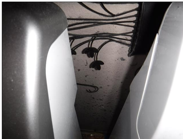
8.4 LAUNDRY/DRYER VENT Item 1(Picture)
