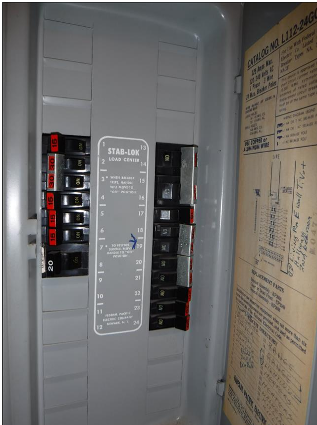
6.2 DISTRIBUTION PANEL Item 2(Picture)
